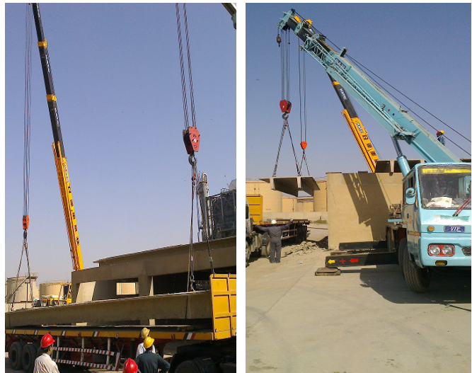
Ware House Shifting for Tee Planks
