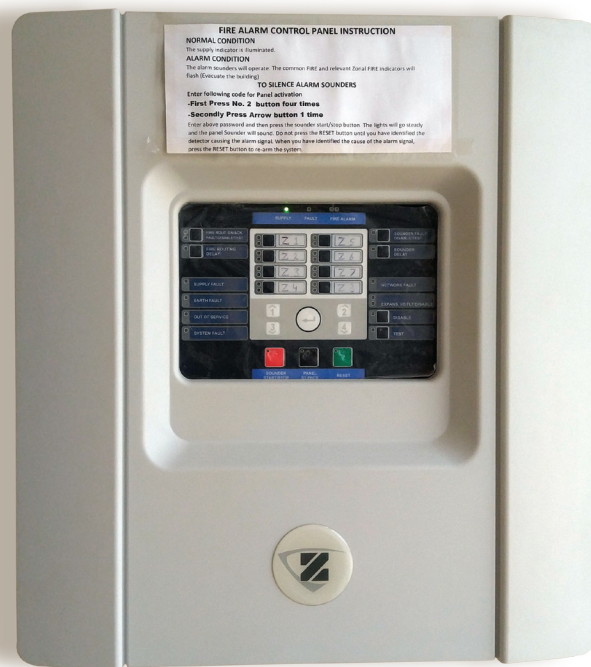
FIRE ALARM CONTROL PANEL
