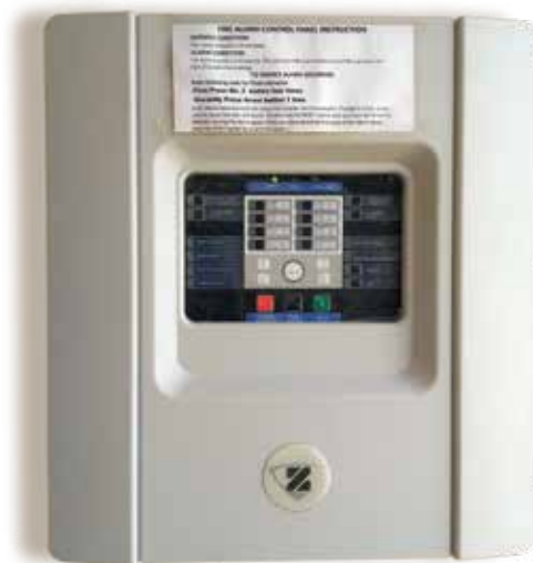
FIRE ALARM CONTROL PANEL
